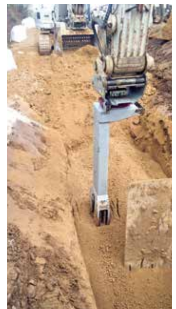
Cable and pipe laying
